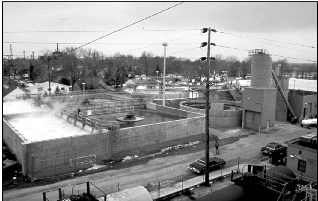
Photograph of water treatment plant on Lake Michigan courtesy of the US EPA.
